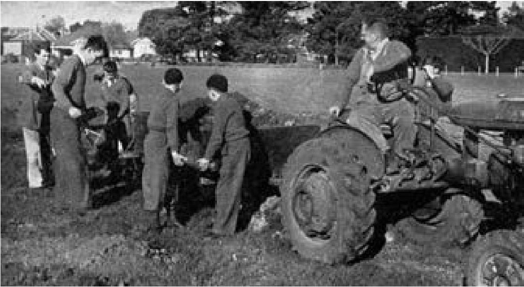
Drainage Operations on the Senior Oval.
